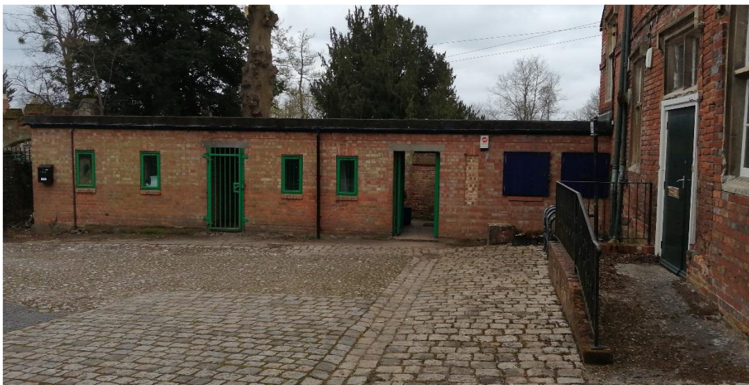
Elevation of southern wing of stable block - location of proposed toilet
