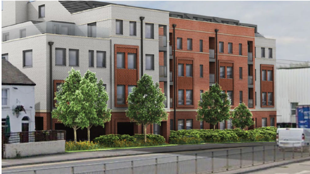
Fig 12 - Individual private entrances and a communal entrance.
