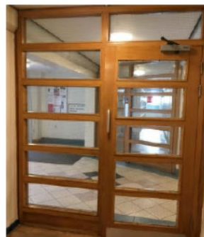
2 - View into entrance lobby
